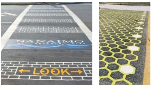
DuraTherm street print allows patterns and logos to be imprinted into crosswalks
